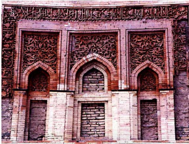
3 Detail of the principal façade, Il Arslan Mausoleum, Urgench, Khwarazm, Turkmenistan
