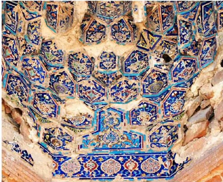
31 Exterior muqarnas vault decorated with mosaic-faience, Mausoleum of Tura Beg Khanum, Urgench, Khwarazm, Turkmenistan
