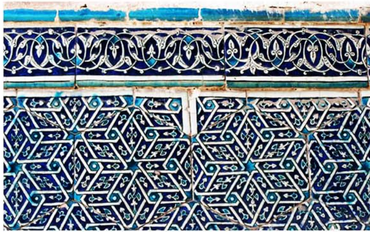
16 Underglaze-painted low-relief tilework decoration on the side of the portal, Mausoleum of Najm al-Dīn Kubrā, Urgench, Khwarazm, Turkmenistan
