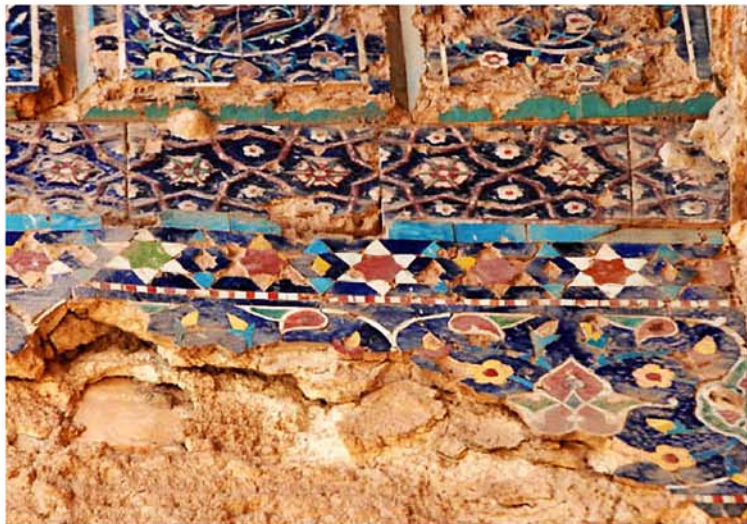
33 Mosaic-faience and cuerda seca tilework decoration inside the portico, Mausoleum of Tura Beg Khanum, Urgench, Khwarazm, Turkmenistan
