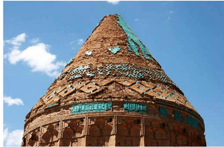
6 The roof of the Tekish Mausoleum, Urgench, Khwarazm, Turkmenistan
