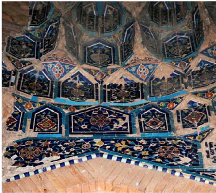
45 Detail of domed vestibule with suspended muqarnas with mosaic-faience, Mausoleum of Tura Beg Khanum, Urgench, Khwarazm, Turkmenistan
