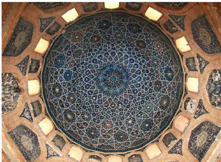
48 Interior of the dome decorated with mosaic-faience, Mausoleum of Tura Beg Khanum, Urgench, Khwarazm, Turkmenistan
