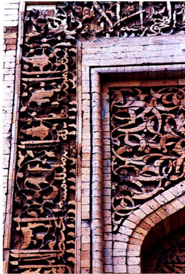
4 Detail of the carved brick panels of the principal façade, Il Arslan Mausoleum, Urgench, Khwarazm, Turkmenistan
