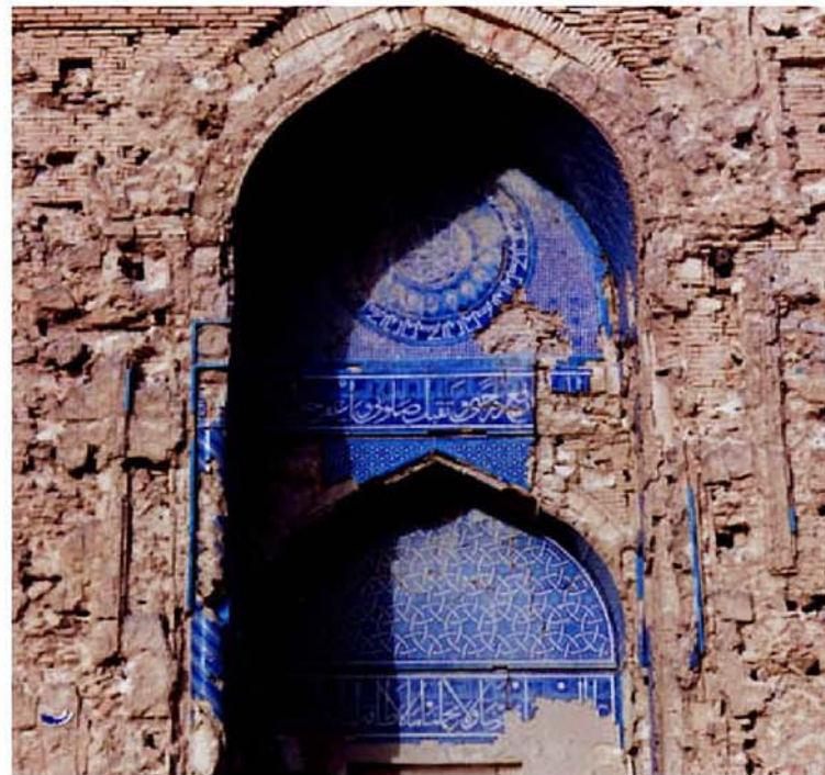
38 Circular medallion in mosaic-faience above the entrance in the portal niche, Mausoleum of Abū Saʿīd ibn Abī 'l Khayr Mayhanī, Mayhana (Meana), northern Khorasan, Turkmenistan (photograph, 2001)
