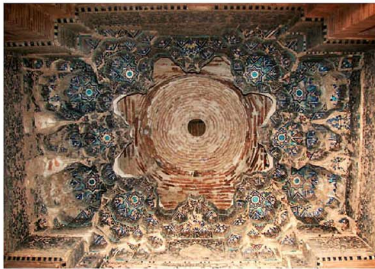
46 Domed vestibule with suspended muqarnas revetted with mosaic-faience, Mausoleum of Tura Beg Khanum, Urgench, Khwarazm, Turkmenistan
