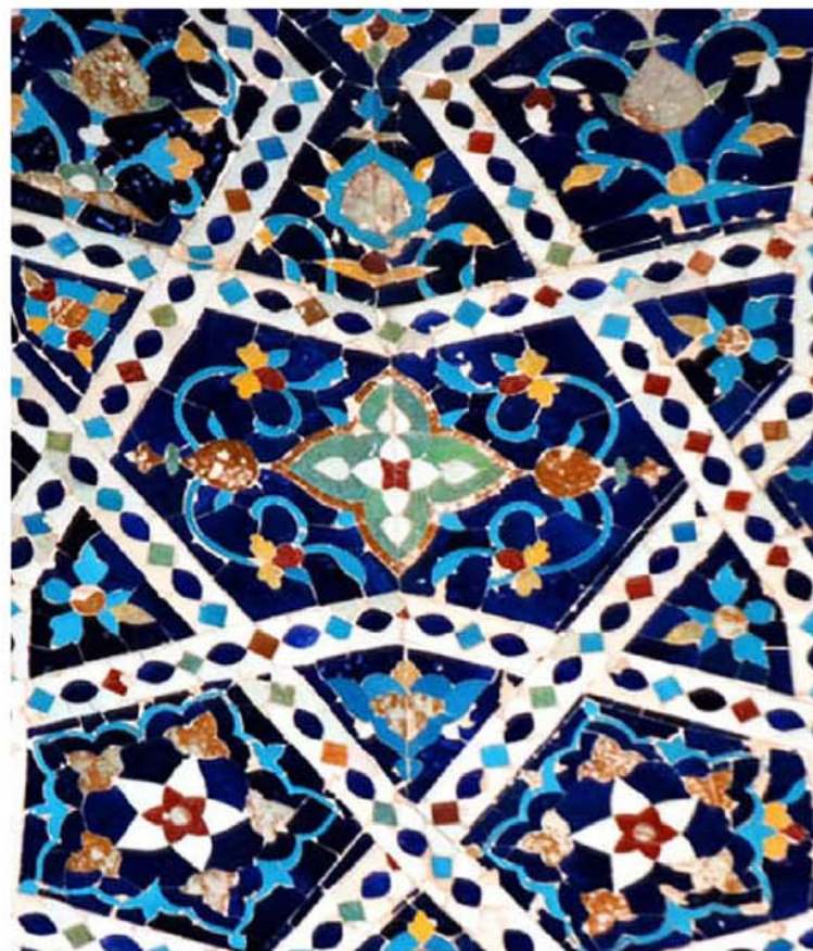
51 Detail of the interior of the dome decorated with mosaic-faience, Mausoleum of Tura Beg Khanum, Urgench, Khwarazm, Turkmenistan
