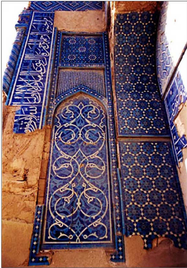
40 Mosaic-faience revetment on the side of the portico, Mausoleum of Abū Saʿīd ibn Abī 'l Khayr Mayhanī, Mayhana (Meana), northern Khorasan, Turkmenistan (photograph, 2001)
